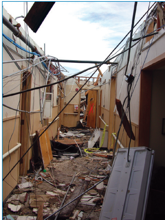
Figure 4-142: View of a main corridor in the 1982 addition
