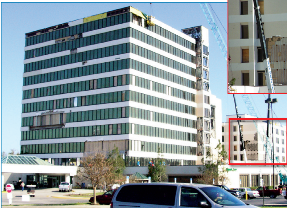
Figure 4-19: EIFS debris blown off the hospital building (Item J on Figure 4-13) in the background (red square) broke numerous windows in the MOB (item G on figure 4-13) in the foreground.
