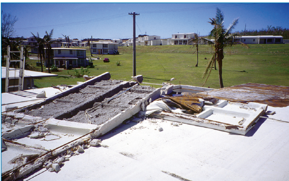
Figure 4-31: Portions of this waffled precast concrete roof deck were blown off. Typhoon Paka (Guam, 1997)
