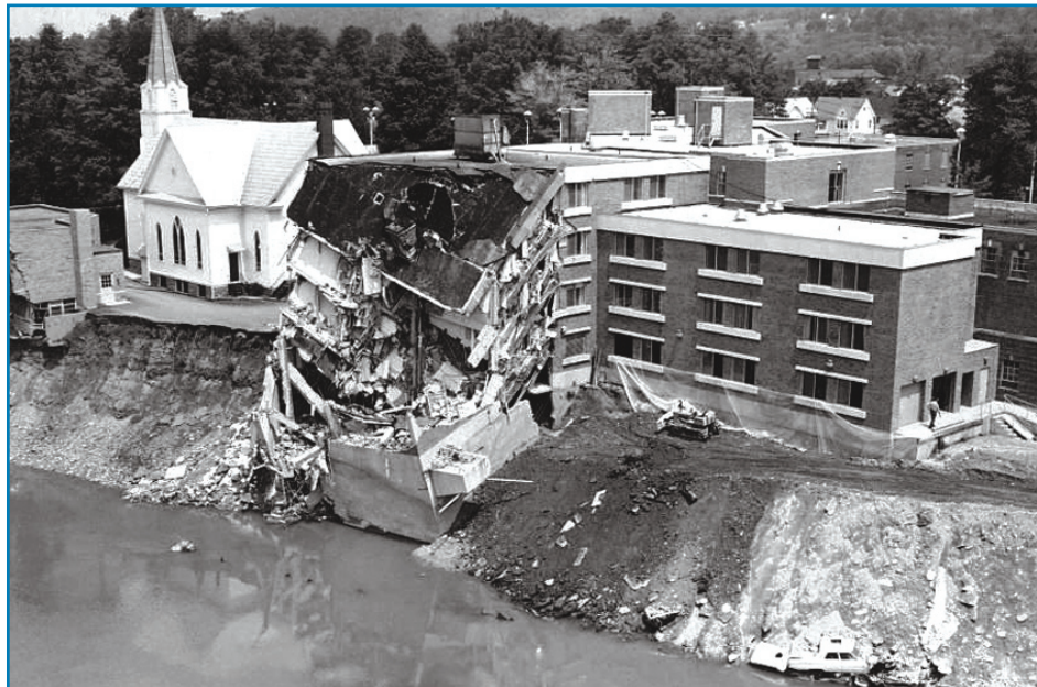
Figure 3-12: Riverbank erosion of the Genesee River during Hurricane Agnes flooding in 1972 eventually led to collapse of this wing of the Jones Memorial Hospital, Wellsville, NY.
