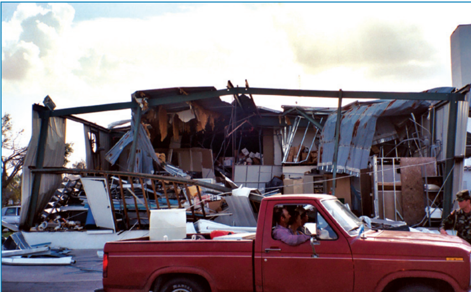
Figure 4-84: This pre-engineered storage building contained the hospital supplies and maintenance shop.
