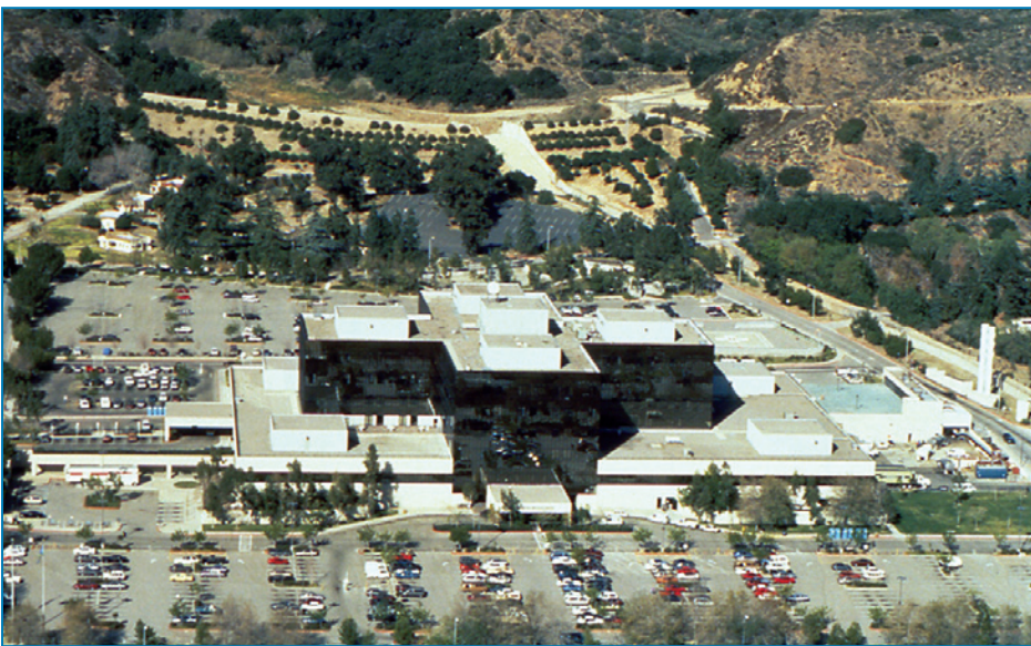
Figure 2-31: Aerial view of “new” Olive View Hospital (1986)
