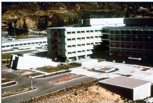
Olive View Hospital After the 1971 Magnitude 6.7 San Fernando Earthquake
