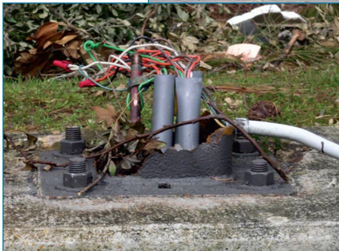
Figure 4-21: Collapsed light fixtures caused by severe corrosion (see inset). The cancer treatment facility is beyond to the left.
